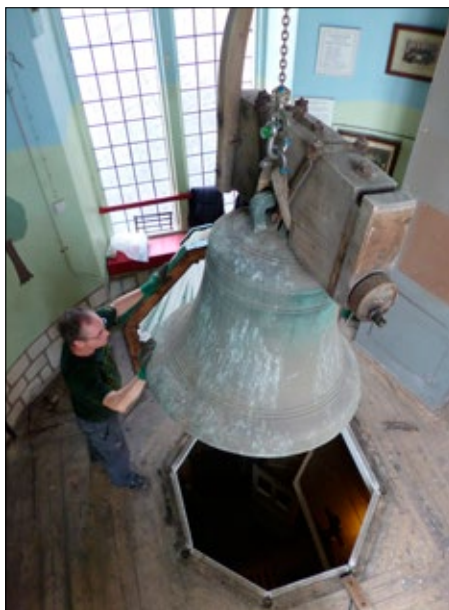
The electric chain hoist broke down with the first bell, so all the bells, fittings and frame parts were lowered by hand. Photos: Dave Kelly / Keltek Trust.
