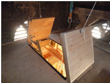
The sound control doors in the new floor above the bell chamber. When open, they let the sound of the bells out. Photo: David Kelly / Keltek Trust.
