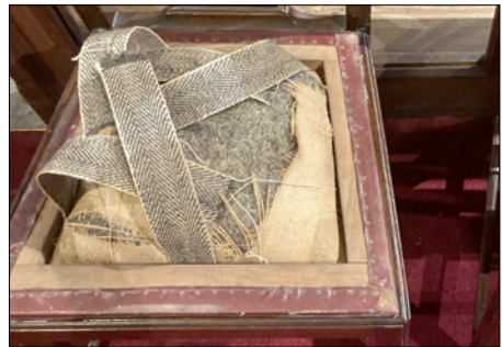
The undersides revealed the original colour – and showed how badly repair work was needed.
